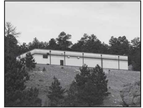
The new rate structure will help make possible large capital improvement projects such as an expansion of the Mary’s Lake Water Treatment Plant.
