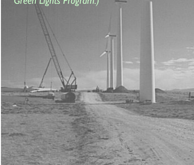
Vestas turbines under construction at the Medicine Bow site.
